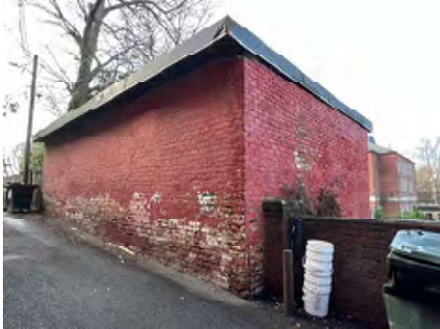
LN0308_114WMainSt_02-2023_AM-085.jpg View SW of E elevation (left) and N elevation (right) of outbuilding, showing two in-filled openings on E elevation
