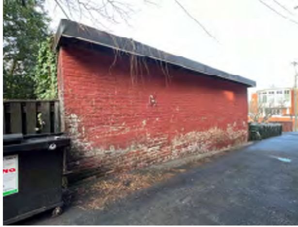
LN0308_114WMainSt_02-2023_AM-086.jpg View NW of E elevation of outbuilding, showing two in-filled openings
